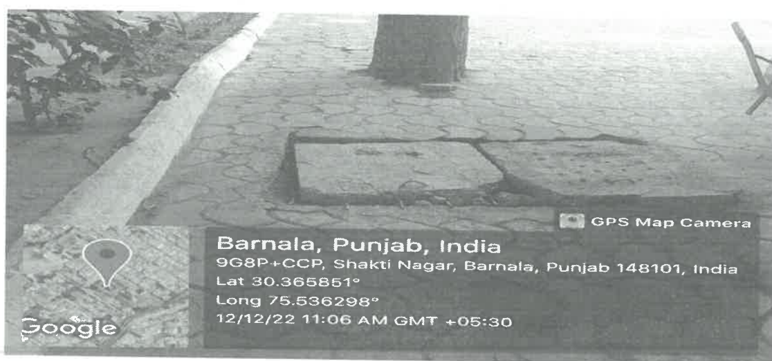
Rain Water Harvesting Pits
