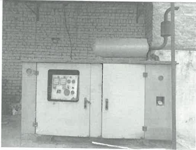
Diesel Generator (15KW+20KW) in the College
