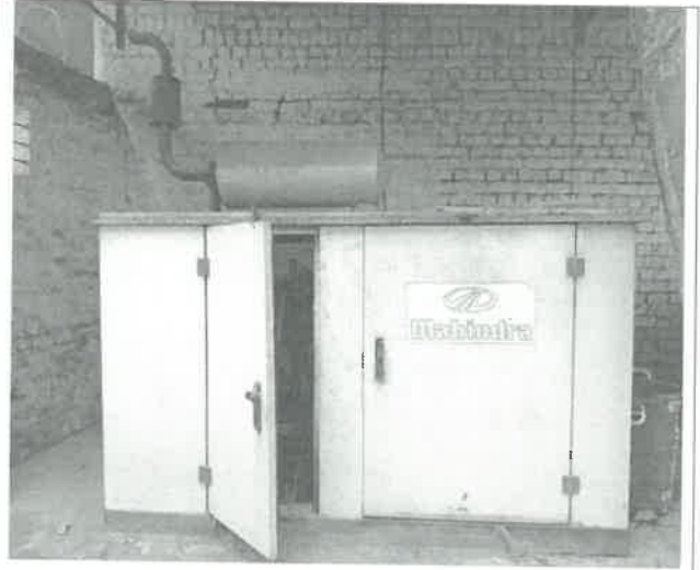
Diesel Generator (15KW+20KW) in the College
