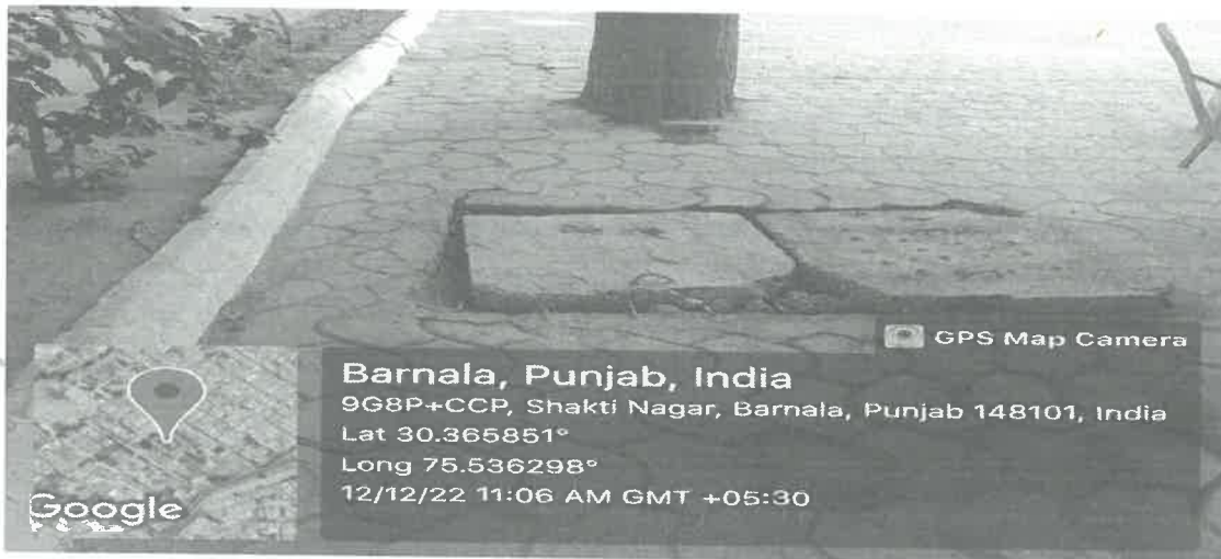
Rain Water Harvesting Pits
