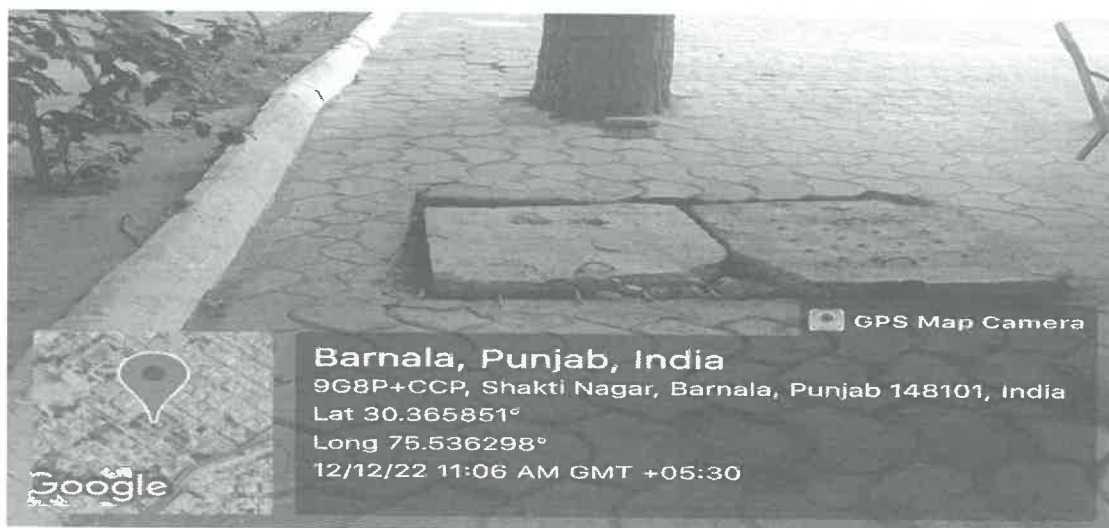
Rain Water Harvesting Pits
